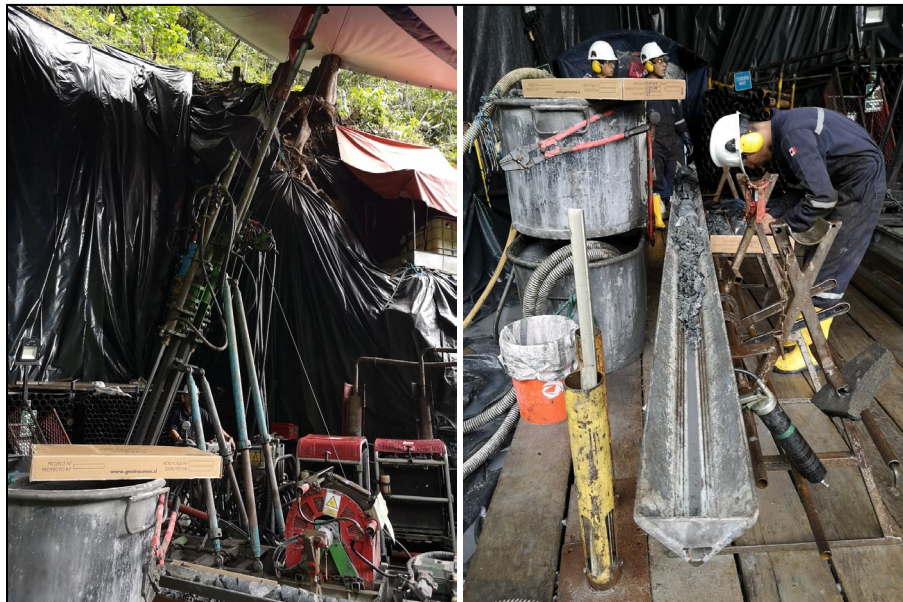
Figure 35: Drilling Platform PE-01, Drill Hole SLSE-08
